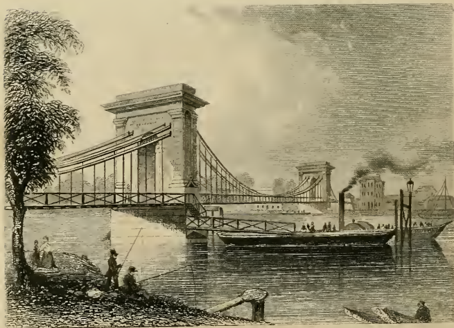
HAMMERSMITH SUSPENSION BRIDGE
